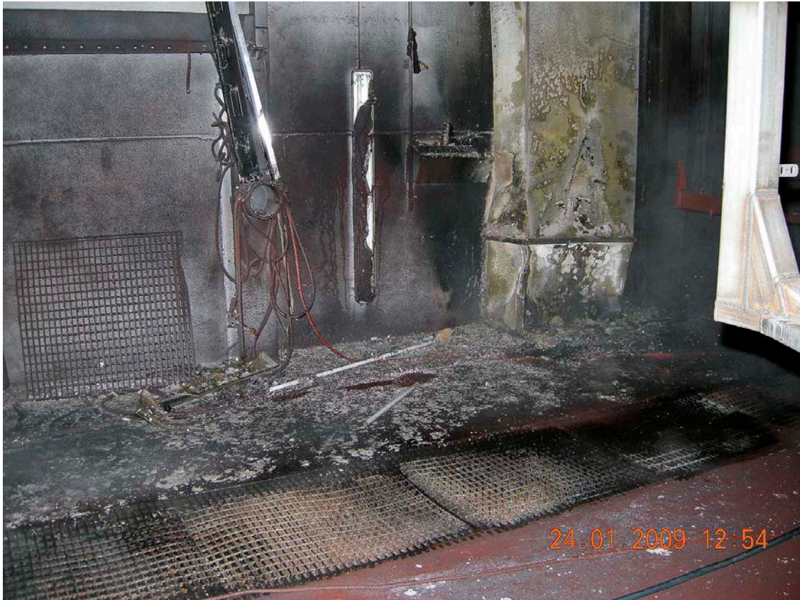
Picture 5 shows where the fire started and the channel through which the fire spread up to the ventilation system.
