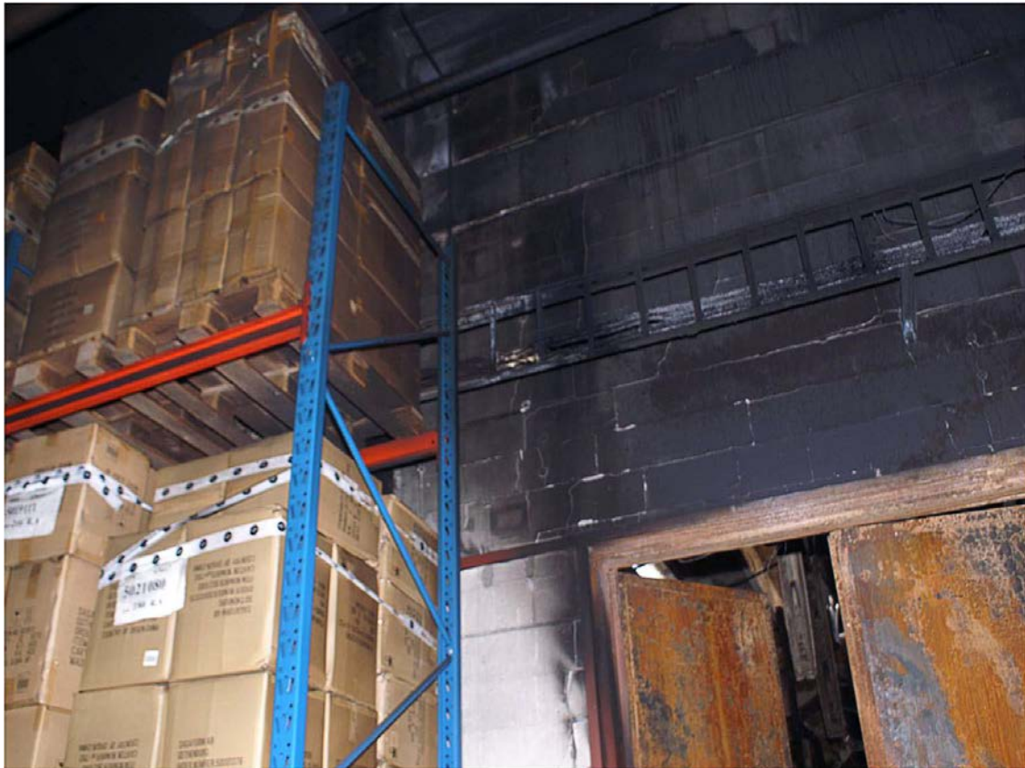
Picture 12 the wall above the door demonstrates clearly that considerable spreading of smoke into the compartment had occurred.
